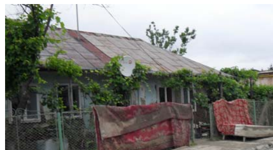
In the photographs on this page one can see the destruction caused by the wall of water, slime, mud and debris after it hit Dorohoi residential dwellings.
